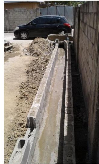
Figure 2: Construction of Box Drains
