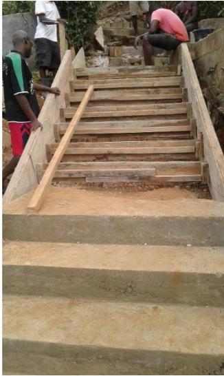
Figure 1: Construction of Stairs in Progress
